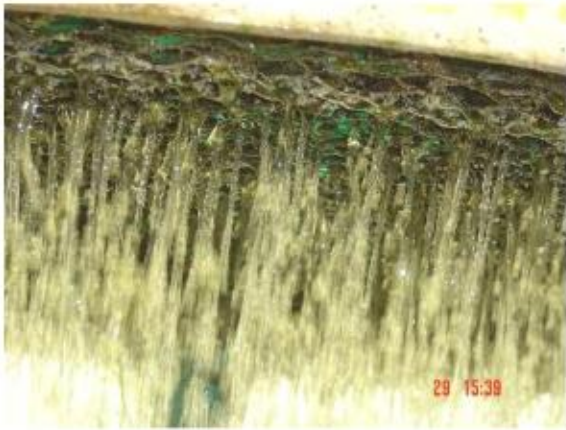
Cooling pad before the installation of the AquaKat
